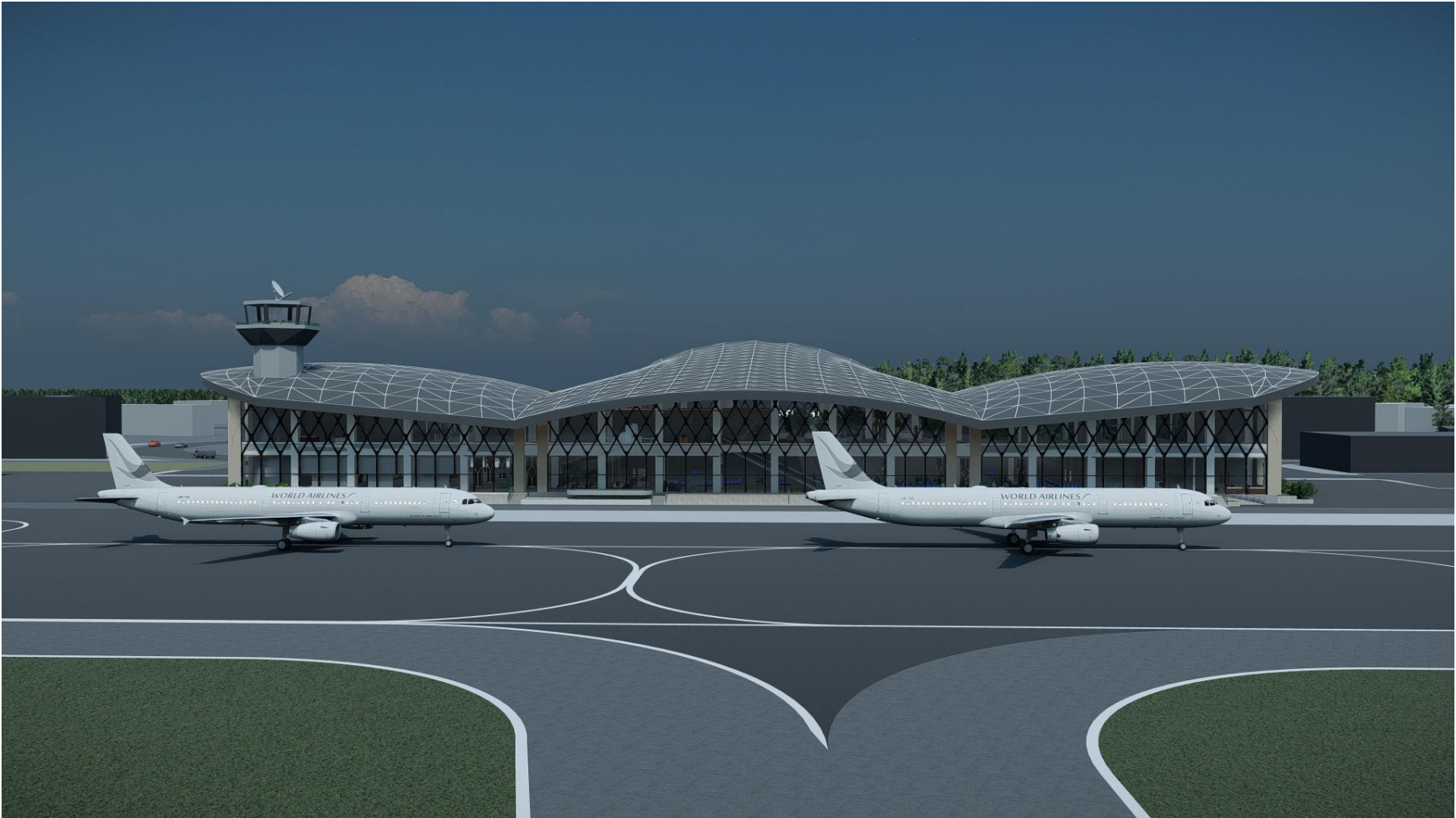
New Terminal Building at Bharatpur Airport
